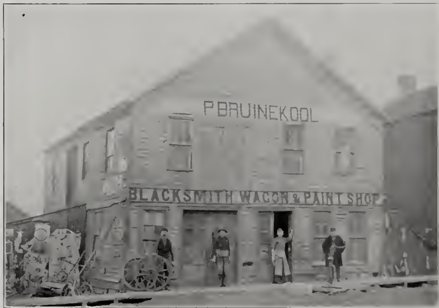
The old Bruinekool blacksmith shop on the west side of the square. A fine brick now occupies its place.
