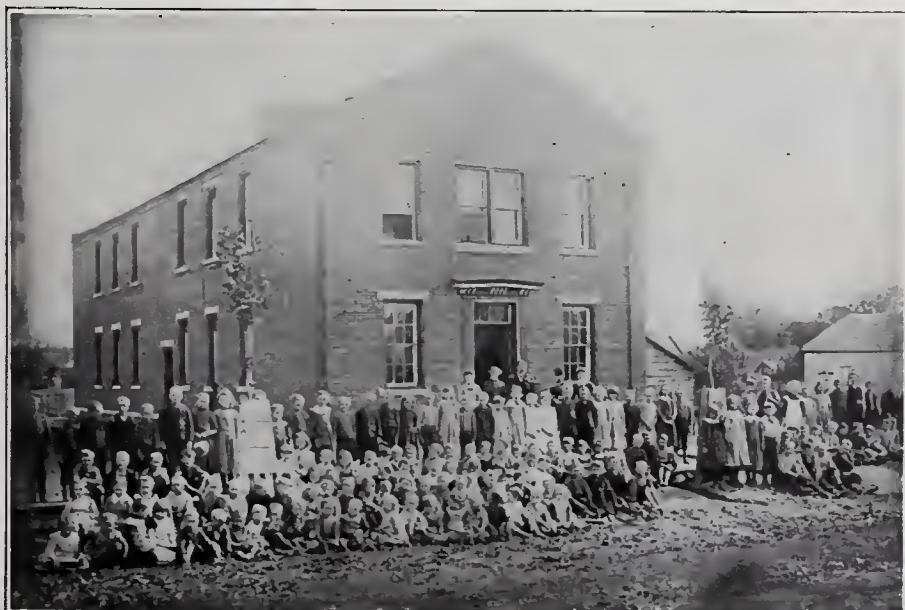
This is the first good school building erected in Pella. The new addition had been built to it in the rear. It was some place then.
