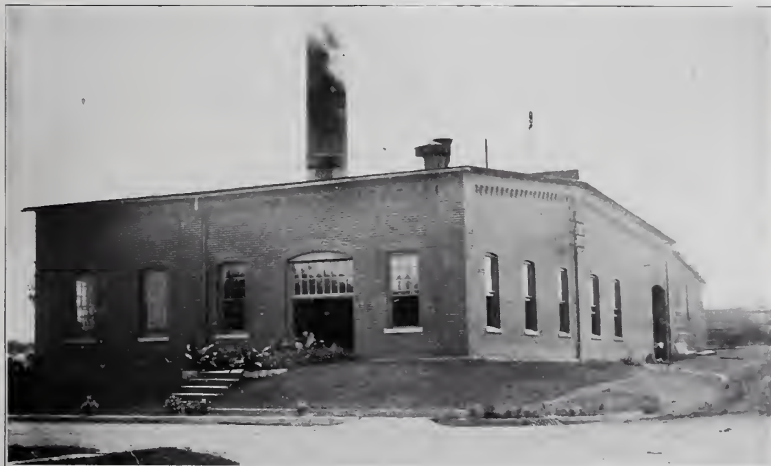
Municipal Light and Power Plant.
