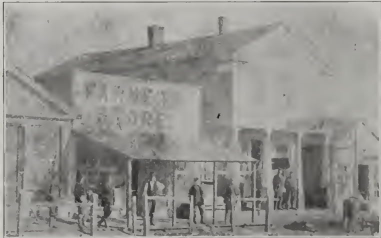
Showing a Portion of the East End of East Franklin Street Between Main and East First Streets
