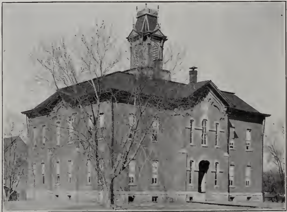
Old Webster School Building
